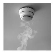
Inside the smoke detector a radioactive source causes ionisation of the air between two electrically charged plates. When smoke enters the detector, the ionisation of the air is reduced.
